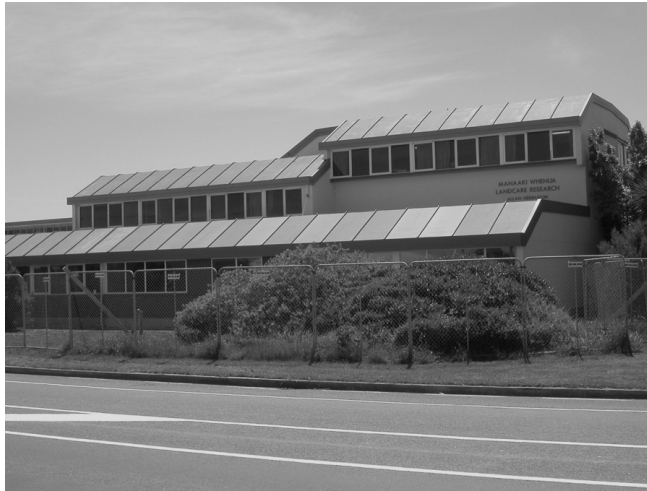
Fig. 3. Exterior of the Allan Herbarium, Lincoln (Nov. 2005, during construction of herbarium addition).
